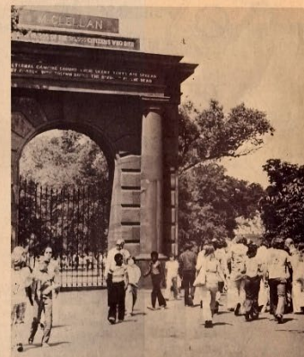
Trudging the Walkways of Arlington
